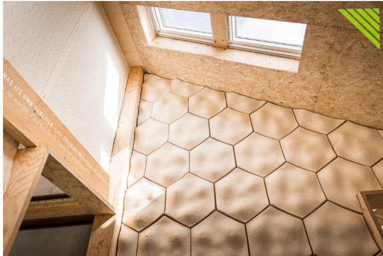
Figuur 4: Mycelium akoestische isolatie. Kamp C, Exploded View Beyond Building ©AR-TUR
